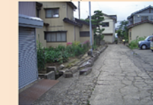
Collapsed concrete-block wall (Mid-Niigata Prefecture Earthquake)
