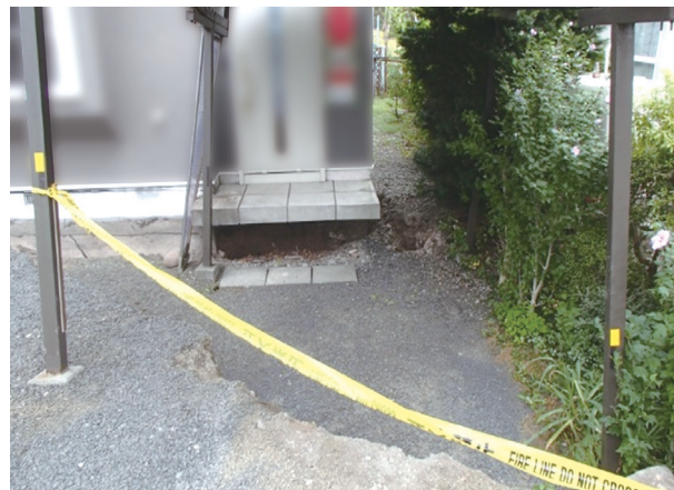
Sinking ground around a building (Hokkaido Bombei East Earthquake)
